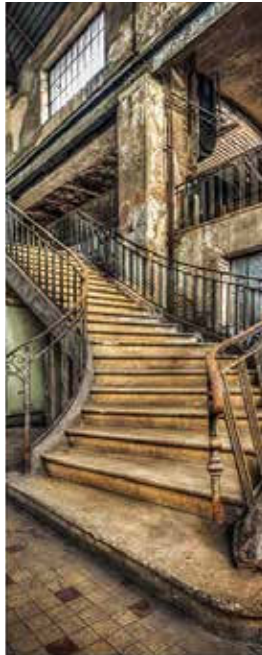
Lost Place - Staircase Prod. Nr. 27589438
