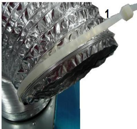
10. Fix the top chimney on the installation bracket (look also on step 8).
